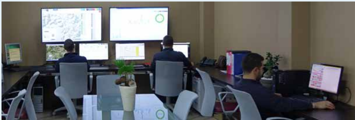
Sardeolica's Control Room
